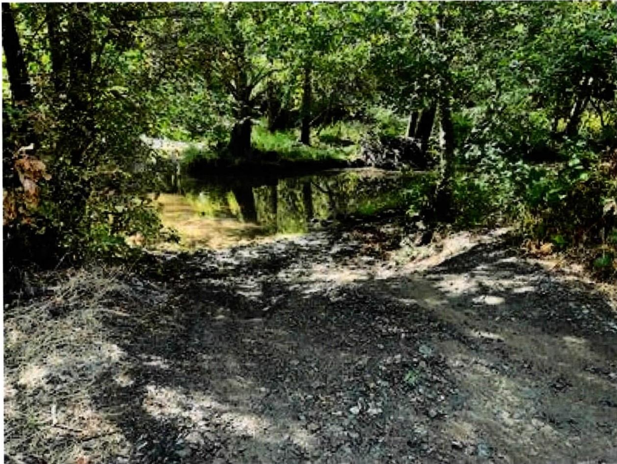
SC-1: Wet ford crossing of Outlet Creek, showing east approach. Fine sediment on the roadway (from both approaches) may pass into the creek, which is a violation of FGC Section 5650.
